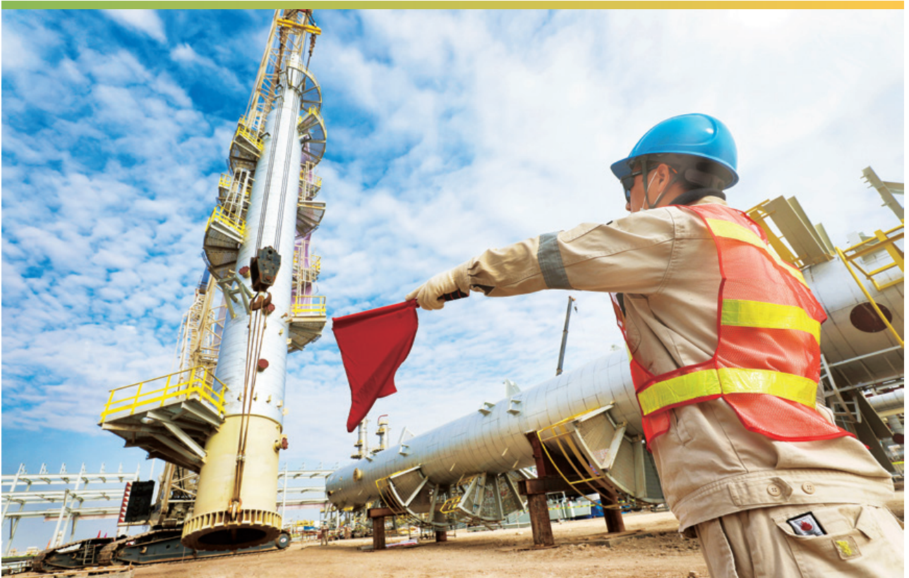
▲ Tower hoisting with a safety supervisor
