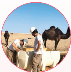
↗ CNPC repairs camel water troughs in Saudi Arabia in line with international standards
