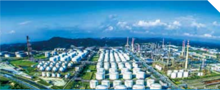
Guangxi Petrochemical invited more than 20 delegates from the surrounding communities to visit the production plant area and the sewage treatment plant, providing them with a face-to-face picture of a green refinery.
