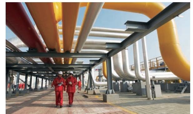
↑ Routine onsite inspection
