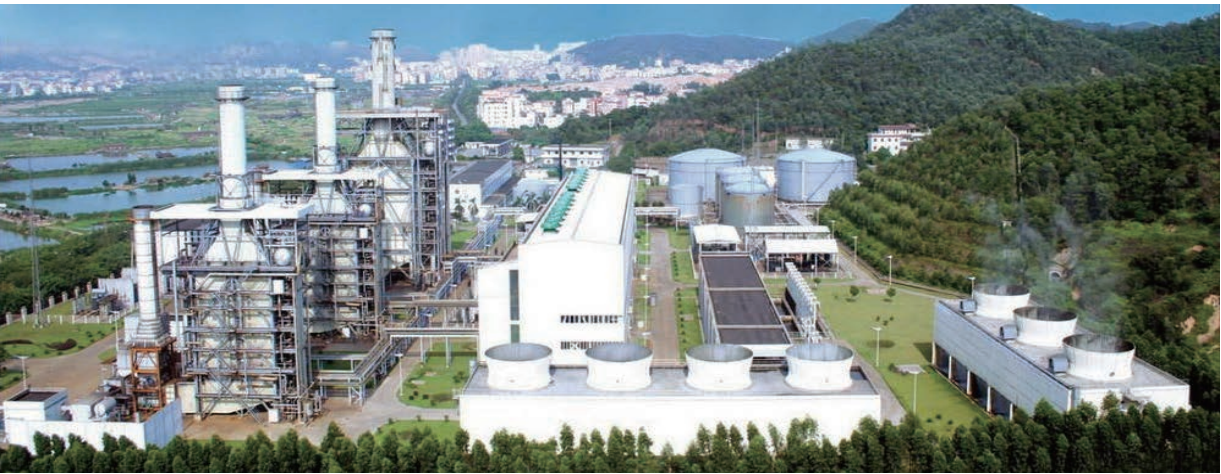
Humen power plant in Guangdong using clean natural gas
