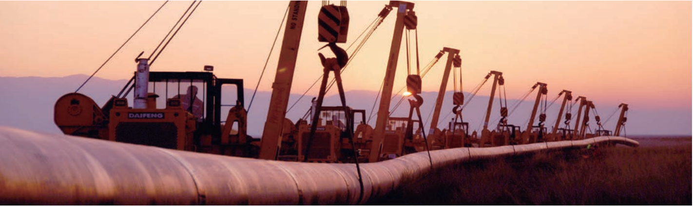
Pipeline laying site
