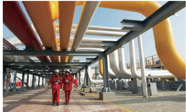
↑ Routine onsite inspection
