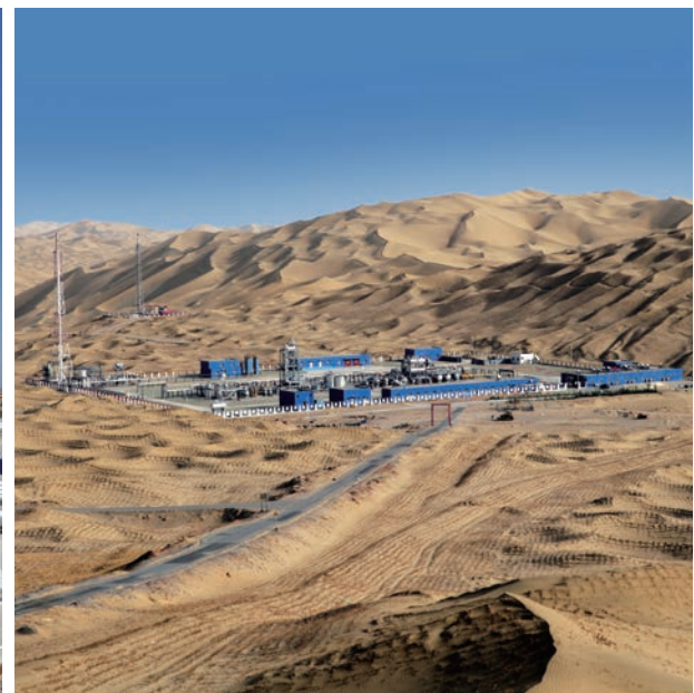
↑ The natural gas plant in the hinterland of the Taklimakan Desert
