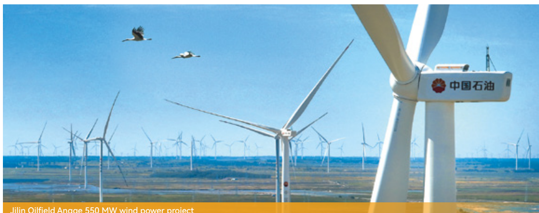
Jilin Oilfield Angge 550 MW wind power project
