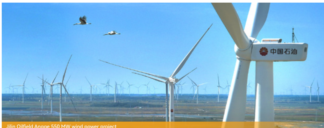
Jilin Oilfield Angge 550 MW wind power project
