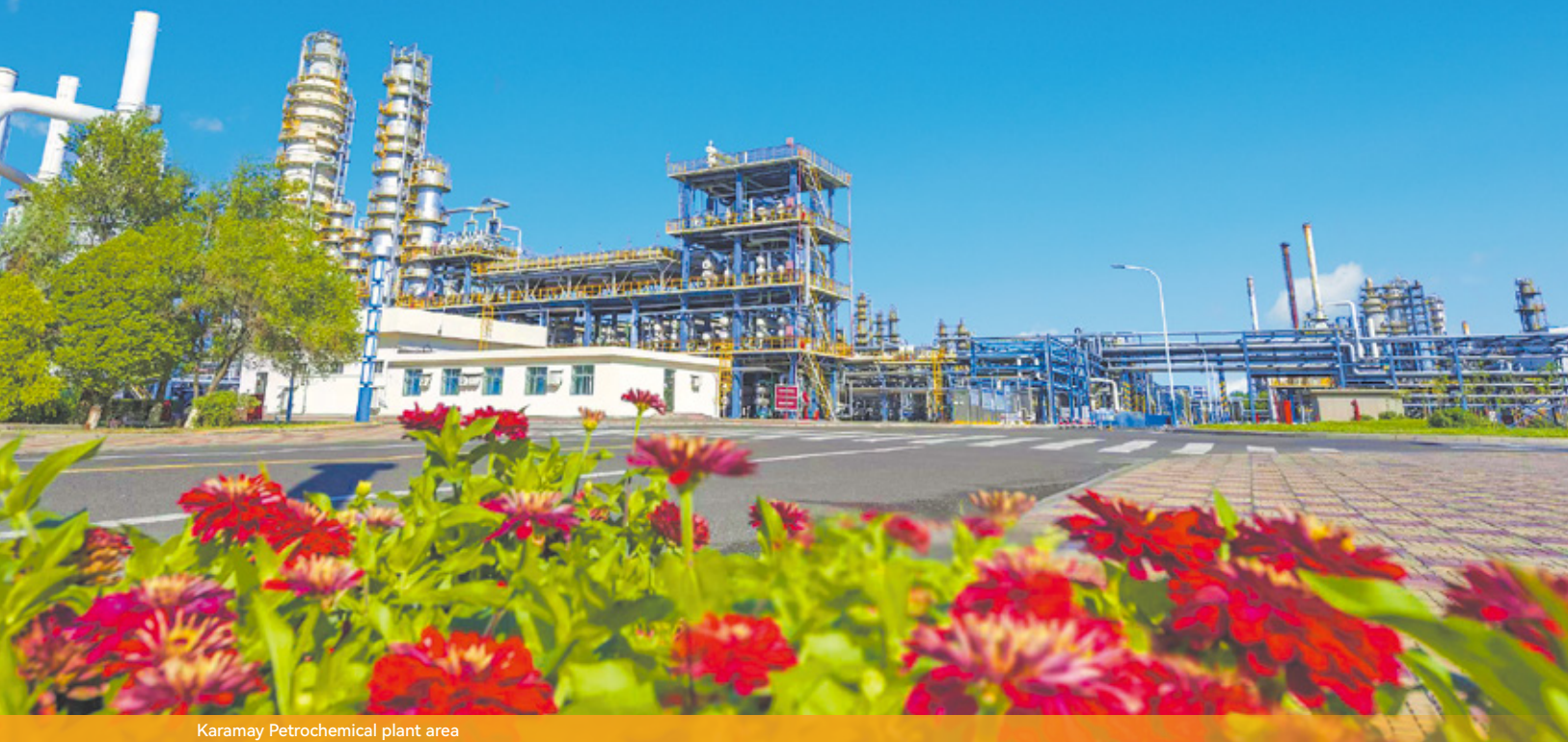
Karamay Petrochemical plant area
