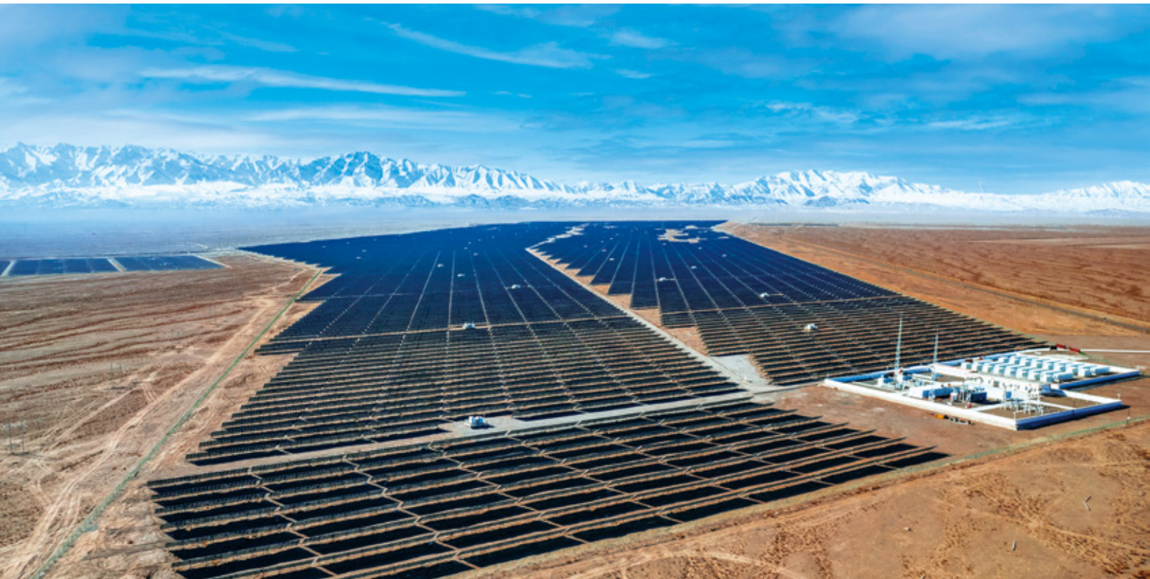
Yumen Oilfield's PV power project
