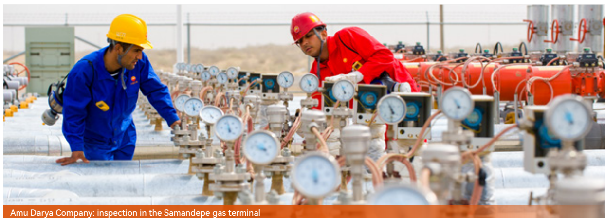
Amu Darya Company: inspection in the Samandepo gas terminal
