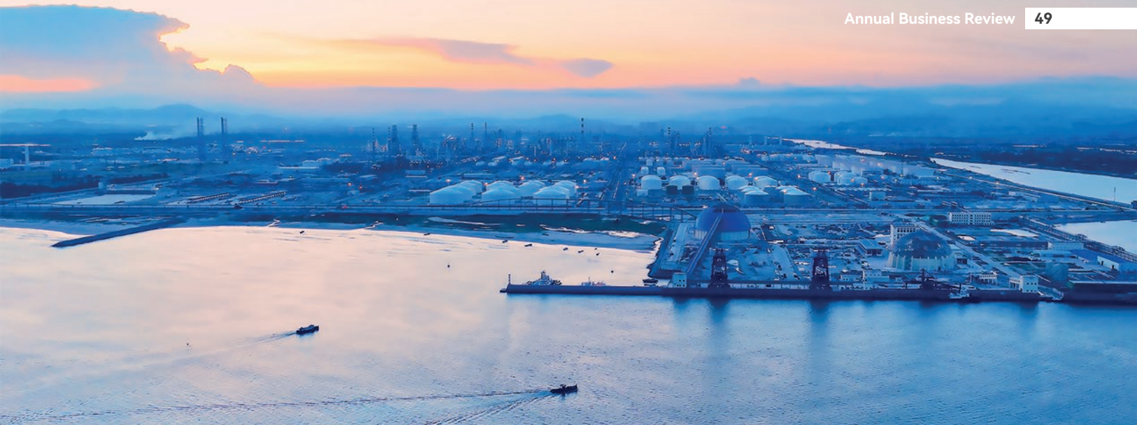
Refining-chemical Integration Project, Guangdong Petrochemical
