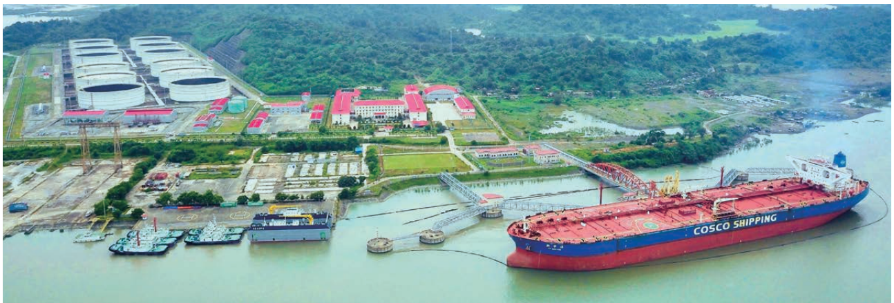
Crude oil jetty on Made Island, Myanmar-China crude oil pipeline
