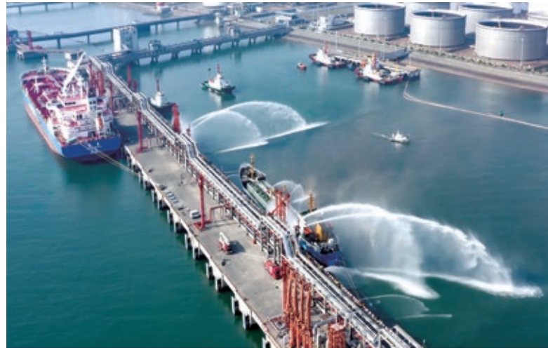
Guangxi Petrochemical conducting emergency drills together with relevant local departments at the 100,000-ton crude oil terminal
