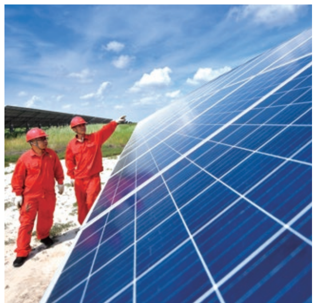
Photovoltaic power generation project at Jilin Oilfield
