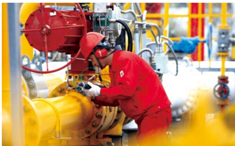
Routing inspection at gas station
