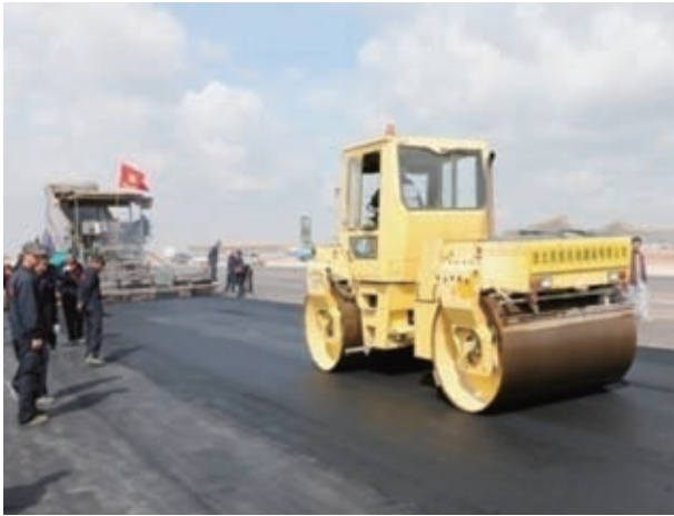
Field application of heavy traffic paving asphalt produced by Venezuelan super heavy oil
