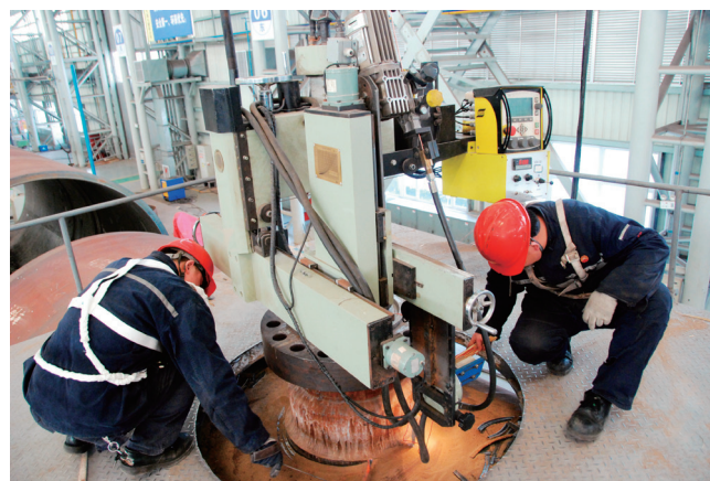
筒身小直径接管马鞍形开口埋弧焊
