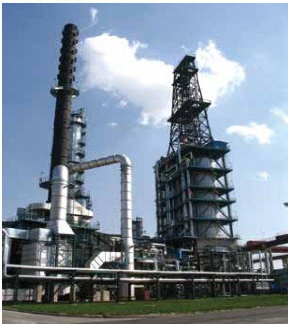
CNPC Liaohe Petrochemical Company's 100×10 4 t/a delayed coker for Venezuela ultra heavy oil residue
