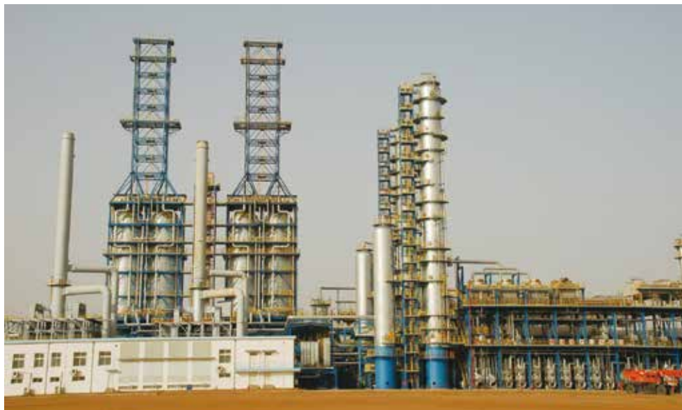
200 \times 10^4 t/a high-acid and high-calcium crude delayed coker in Sudan Khartoum refinery
