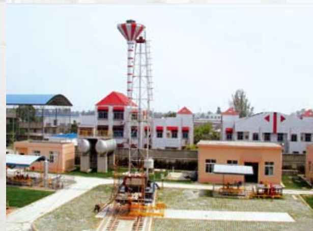
Full view of the simulating experimental system for gas production
