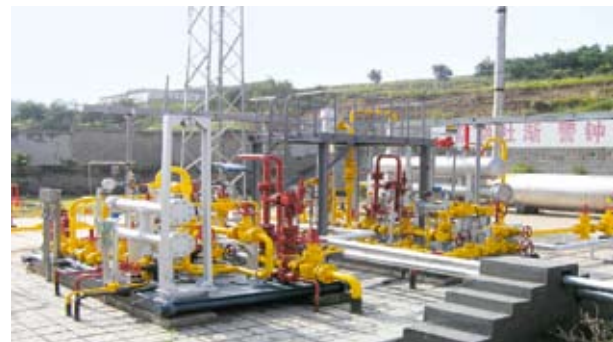
Corrosion test devices in the high sulfur gas field
