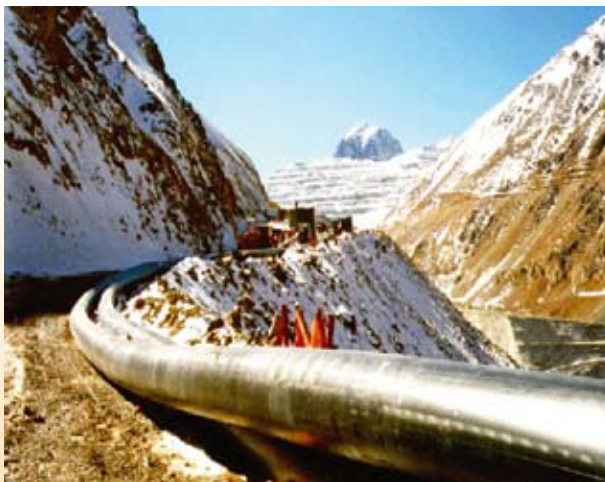
Gas gathering pipeline of gas/liquid miscible transportation system in Yingmai-7 filed
