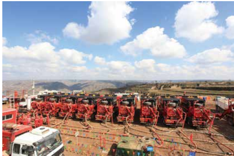
hydrojet fracturing site operation
