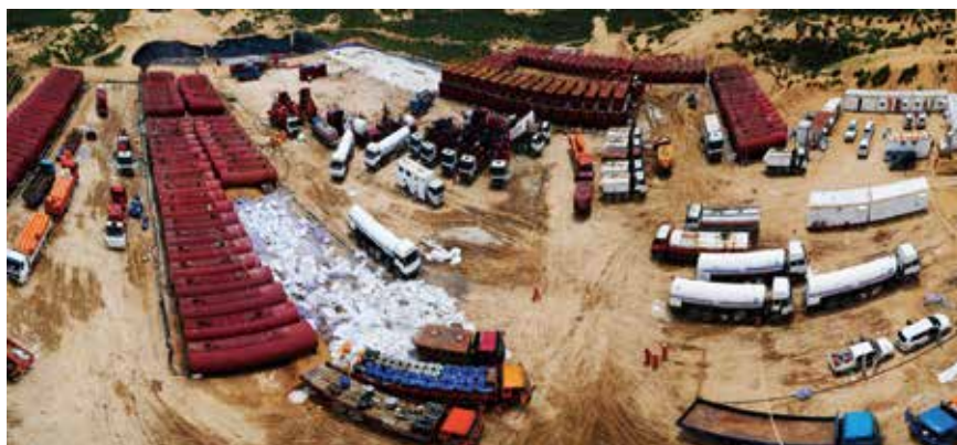
Hydrojet fracturing operation site of well B (gas field)
