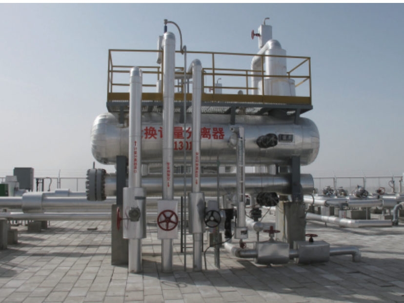
Oil-gas mixing transportation metering separator
