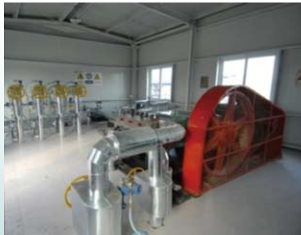
Interior of Injection Station
