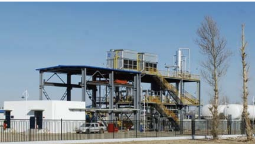
Hei-59 Liquid Gas Injection Station
