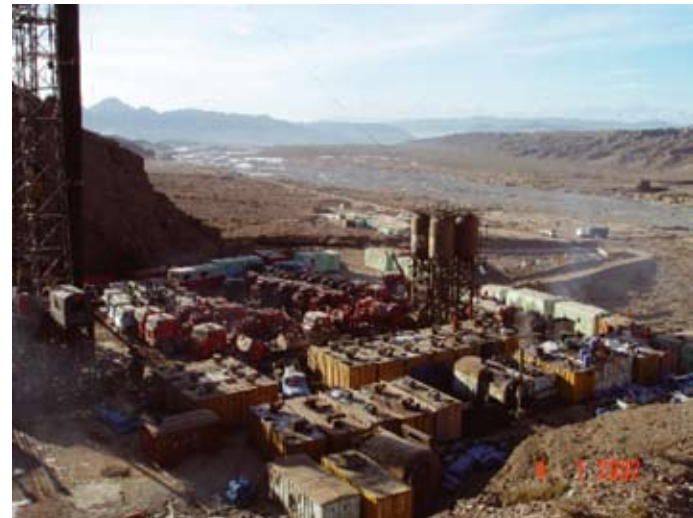
Fracturing Operation Site of Well Ake1 in Tarim
