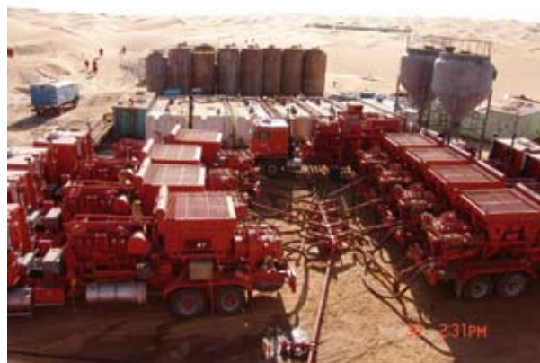
Fracturing Operation Site of Ultradeep Well in Tarim
