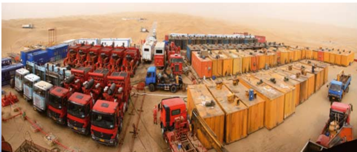
Operation Site of Staged Acid Fracturing Technology for Horizontal Wells (Surface Cross Linking Acid)
