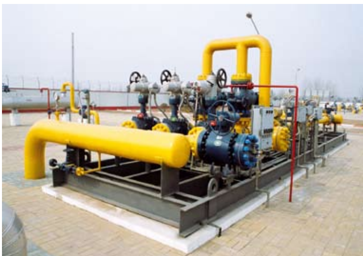
Skid-mounted unit at the station
