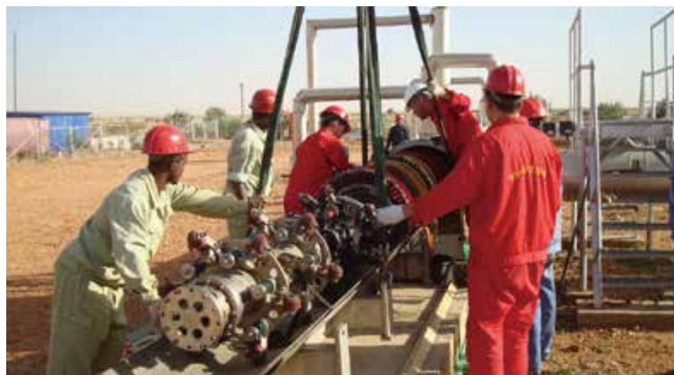
Figure 3-2 Pig launching for intelligent detection of \phi 711 pipeline
