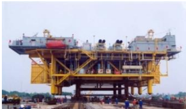
Slide shipment of topside module
