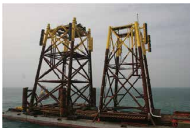
Offshore installation of jacket
