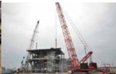
Site general assembling of topside module
