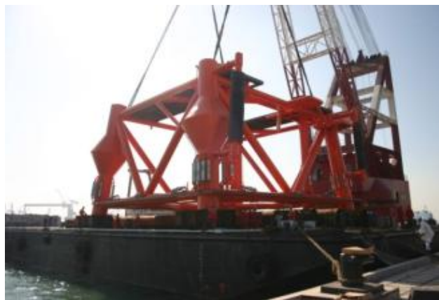
Jacket hoisting and shipment
