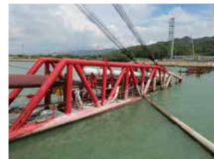
Bottom drag construction in the landing section
