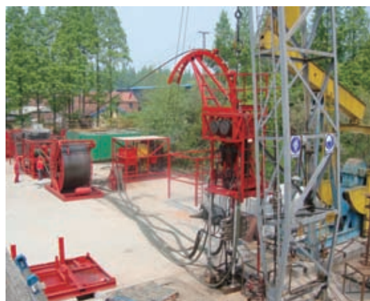
Professional equipment commissioning and field service team
