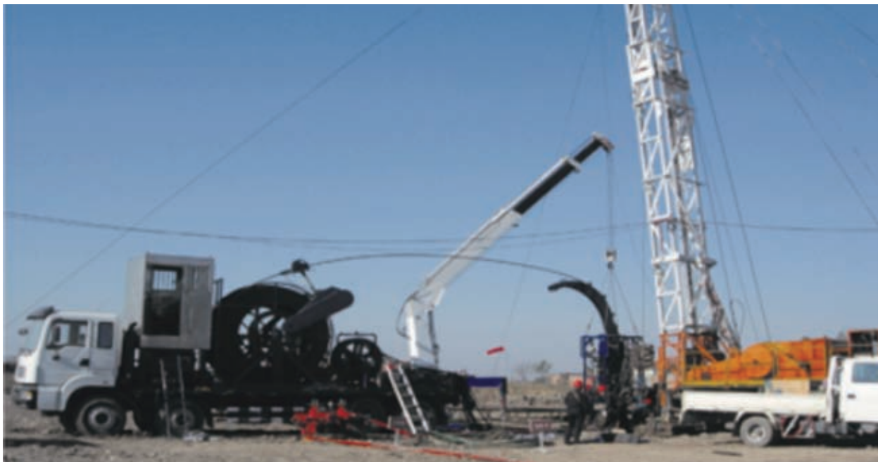
Sand washing and plugging removal operations in well H1 in Dagang Oilfield
