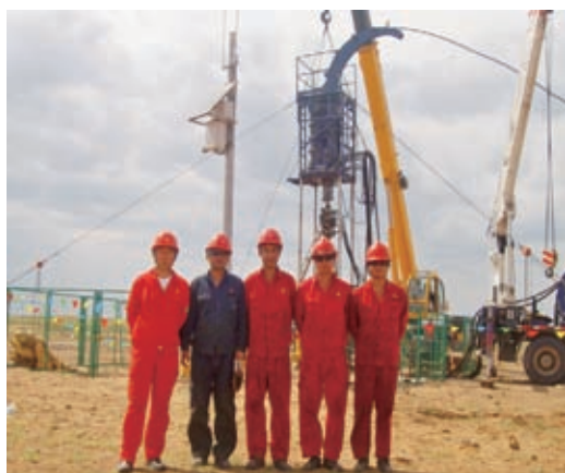
Special-purpose test well site for commissioning of equipment
