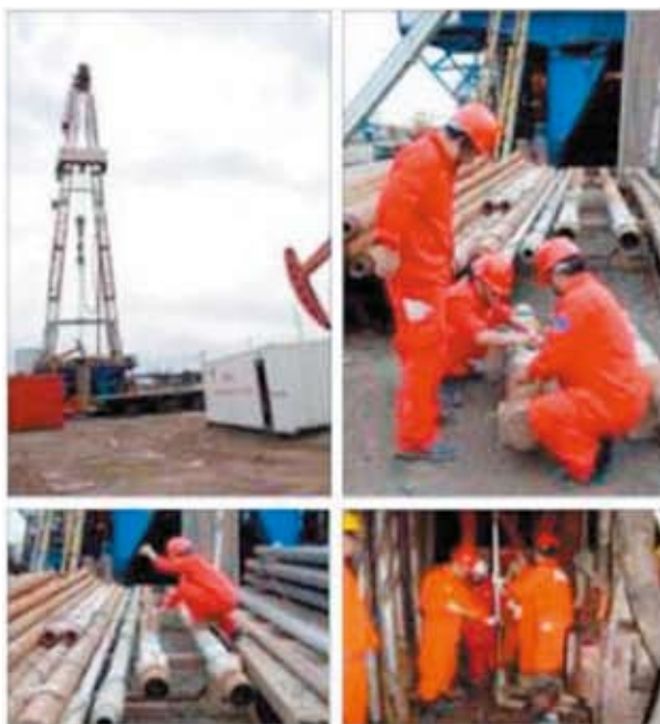
System test is conducted before operation
