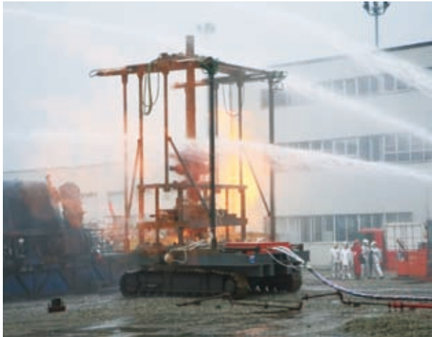
Wellhead reconstruction equipment
