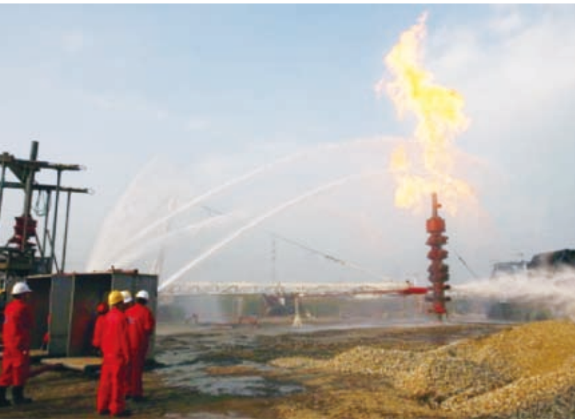
On site treatment of blowout of sour oil and gas well
