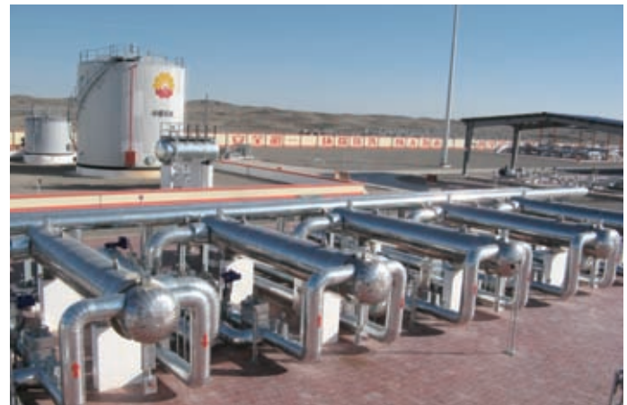
Cyclone separator of second west-east gas pipeline
