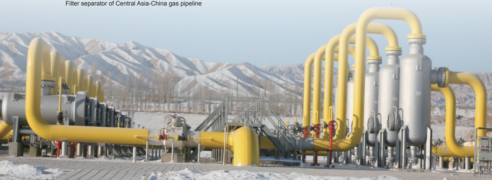
Filter separator of Central Asia-China gas pipeline
